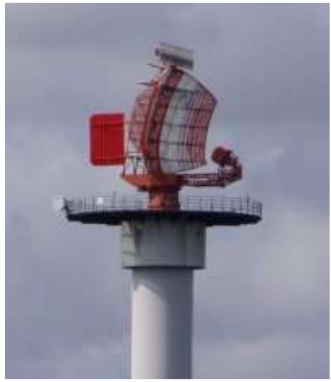
↑ Monopulse Mode S PSR + MSSR
